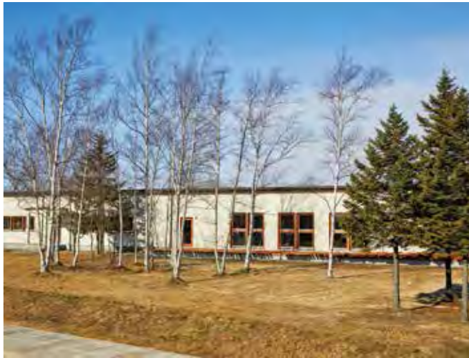
▶ [CTC2] Exterior: Features a terrace.
