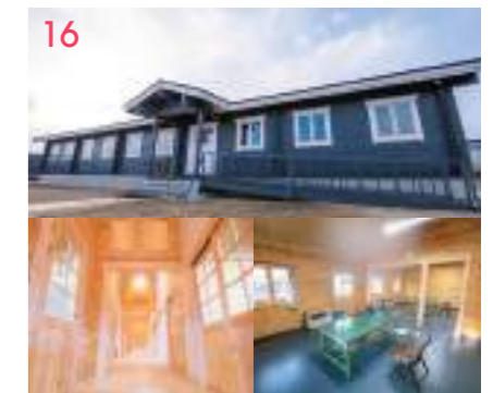
16 Skill Test Building An established proficiency test venue for obtaining a national certification for aircraft mechanics.
