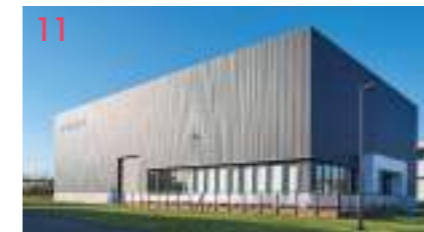
11 Cabin Training Center (CTC) With Airbus A330 and A380 mock-ups installed.
